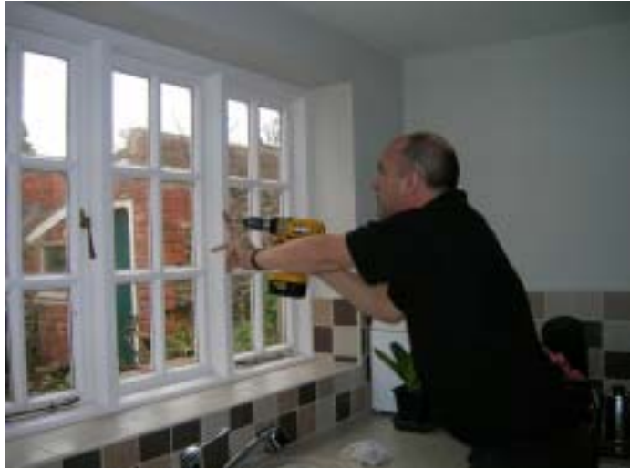
Handy Van Fitter Adam Watson fitting window locks in Diseworth
